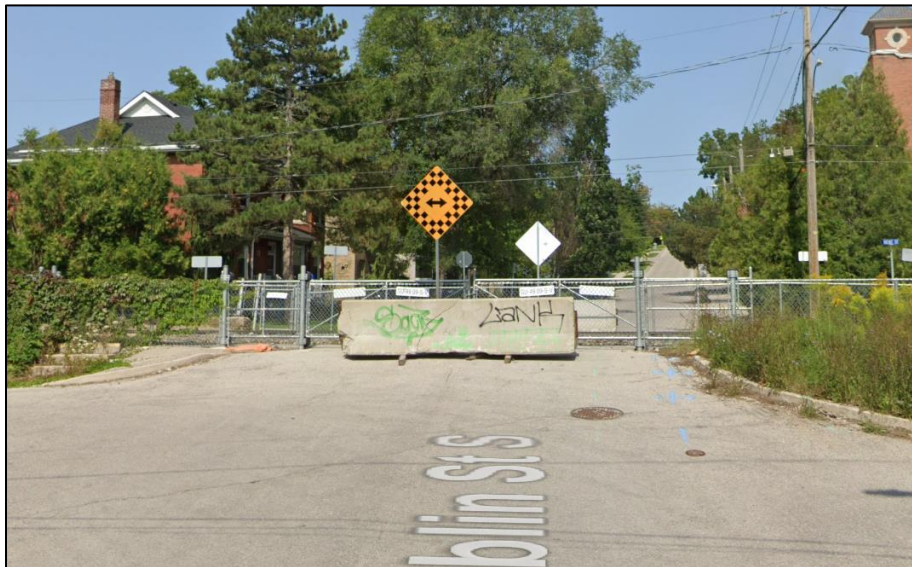
Figure 8 Facing north at the Dublin Street crossing. (Google Maps, 2023)
