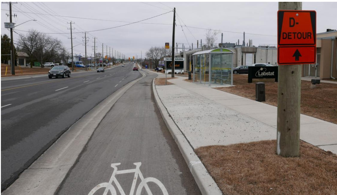
Figure 7-8: Example of Curbside-Bike Lane Stop
