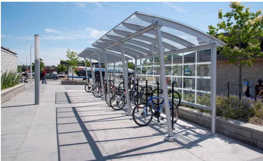
Figure 8-12: Covered Bicycle Parking at an ION Bus Station
