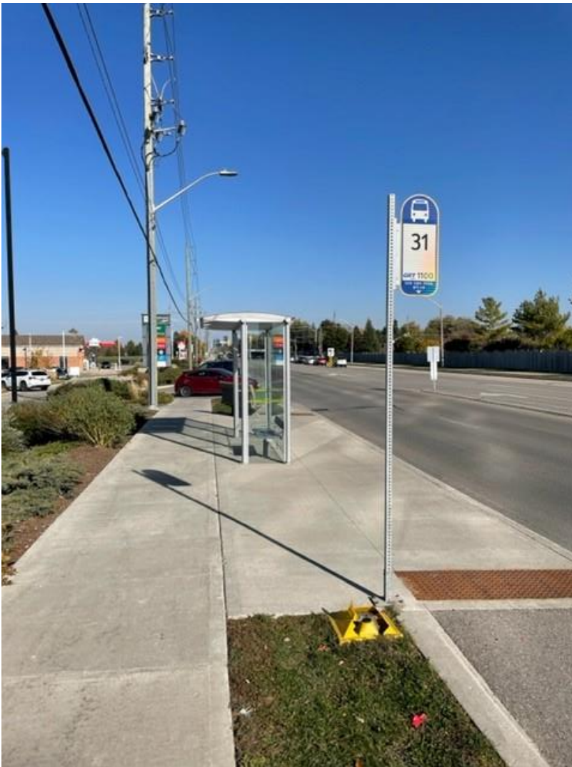
Figure 7-10: Example of Shared Curbside Cycle Track Stop
