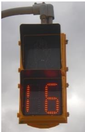
Figure 0-1: Typical Pedestrian Countdown Signal: Typical Pedestrian Countdown Signal
