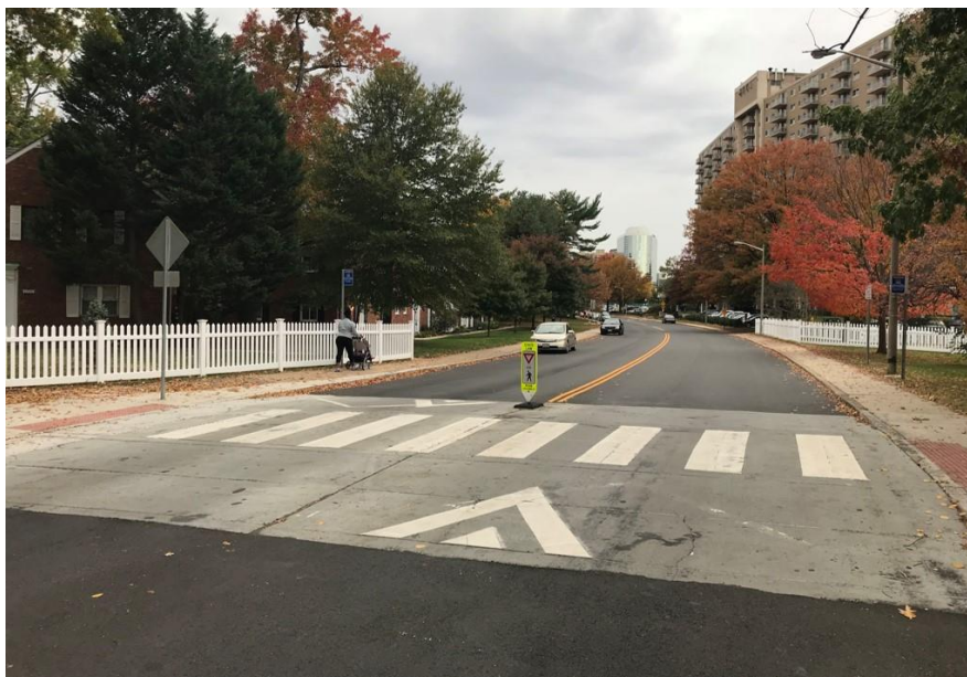
Figure 9: Raised Mid-block Pedestrian Crossing (Source: FHWA)
