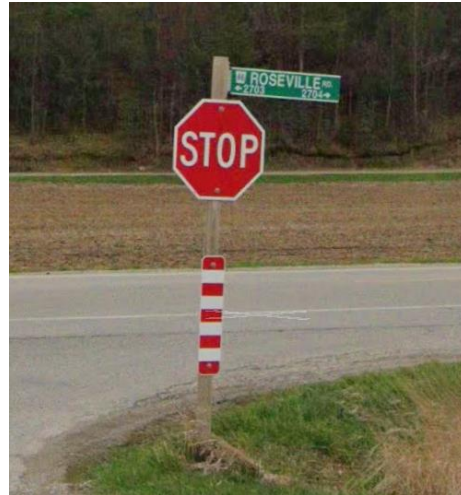
Figure 0-11: Typical Tiger-Tail Sign under a Stop Sign
