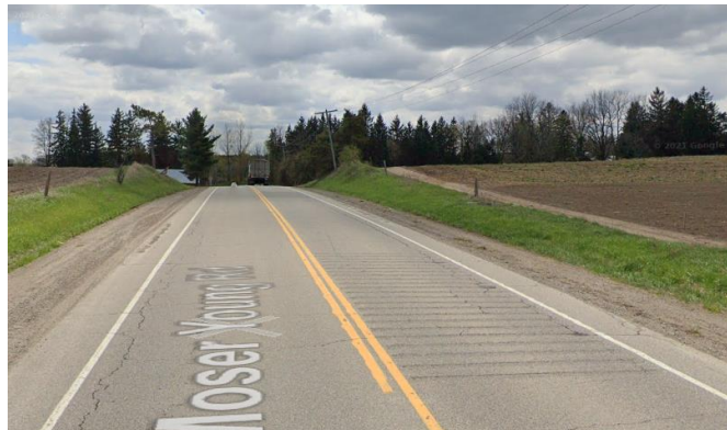
Figure 0-13: Typical Application of Audible Rumble Strips
