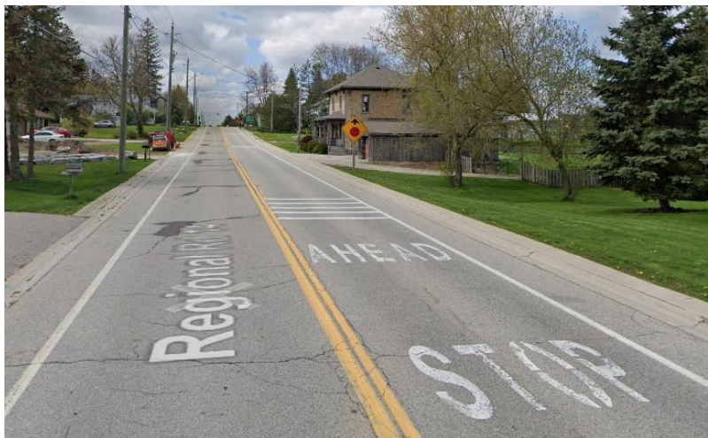
Figure 0-6: Typical Application of Transverse Rumble Strips
