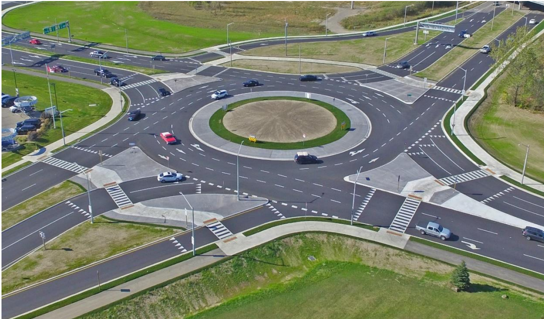
Figure 0-15: Roundabout at Ottawa Street & Homer Watson Boulevard
