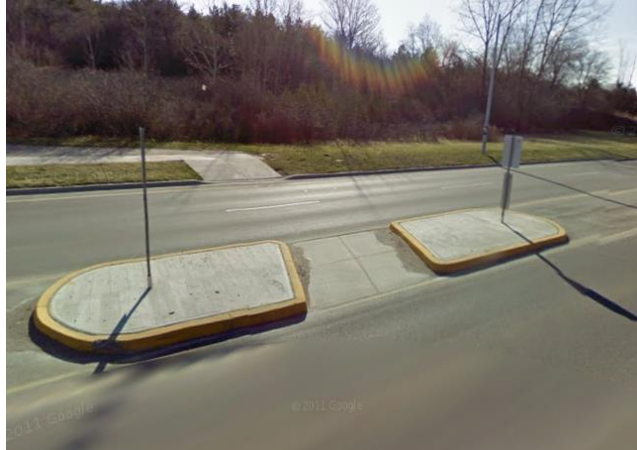
Figure 0-12: Typical Pedestrian Refuge Island
