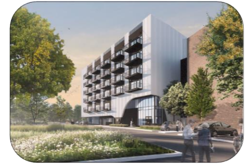
Waterloo Region Housing Revitalization
