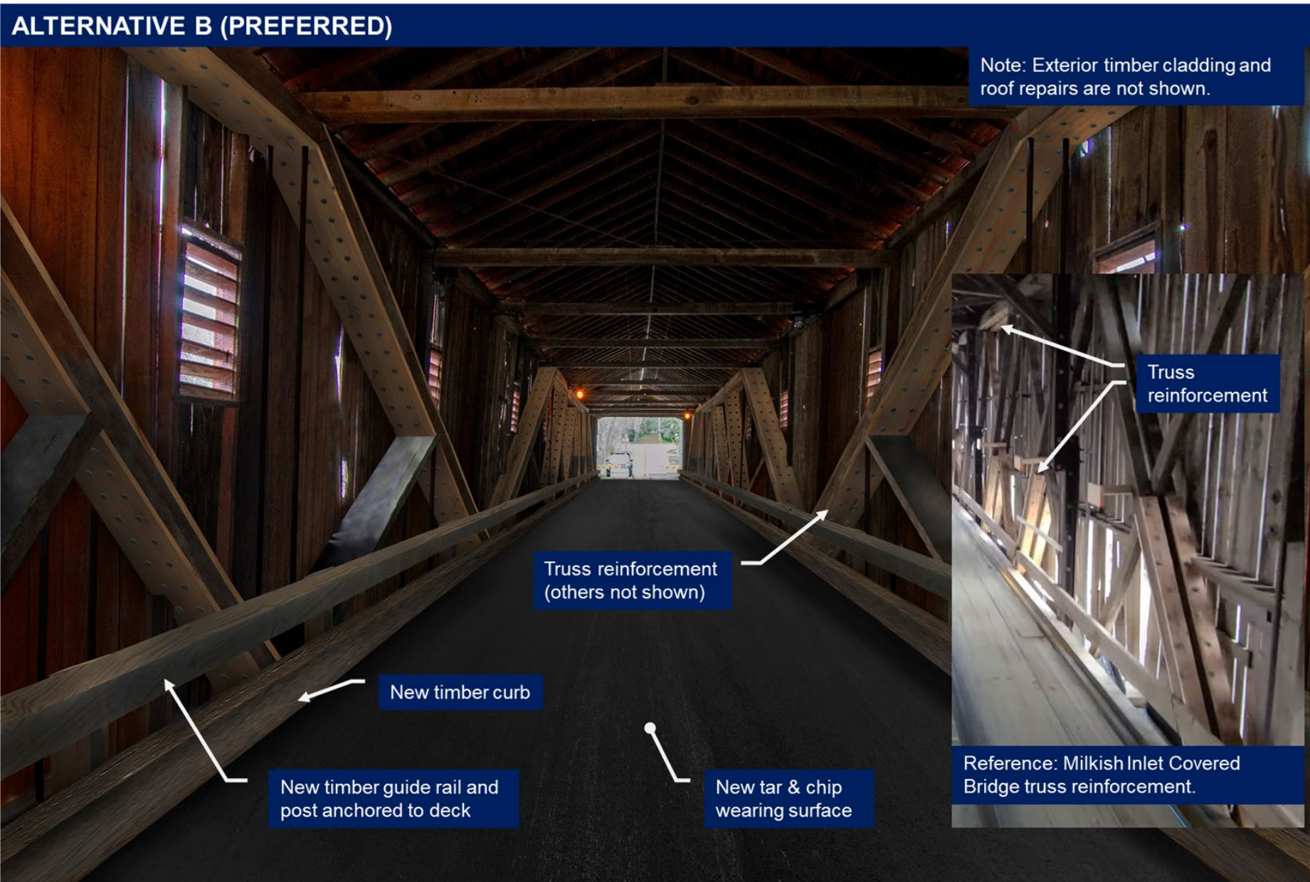
Figure C8: Interior View –Alternative B (Timber Truss Reinforcement)
