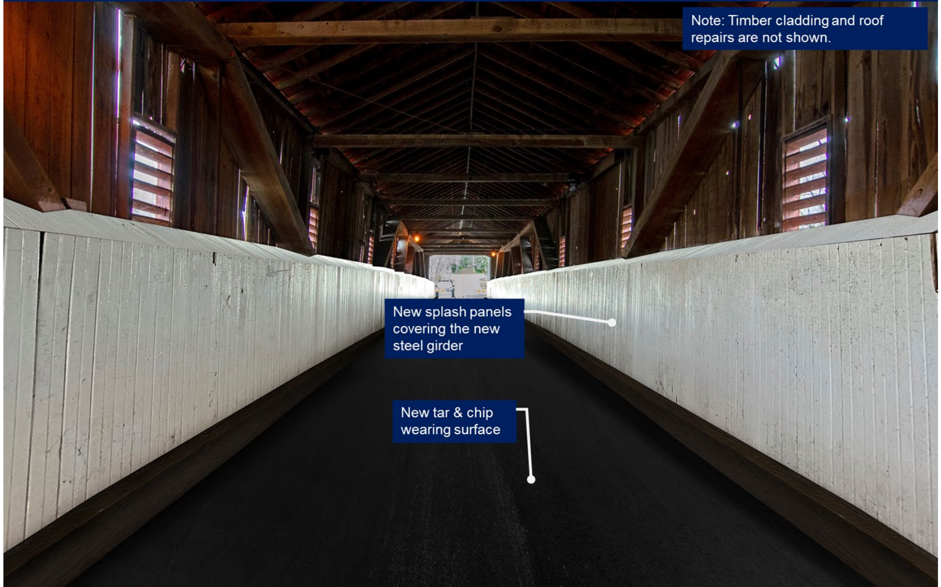
Figure C7: Interior View – Alternative A (Steel Girder Reinforcement)
